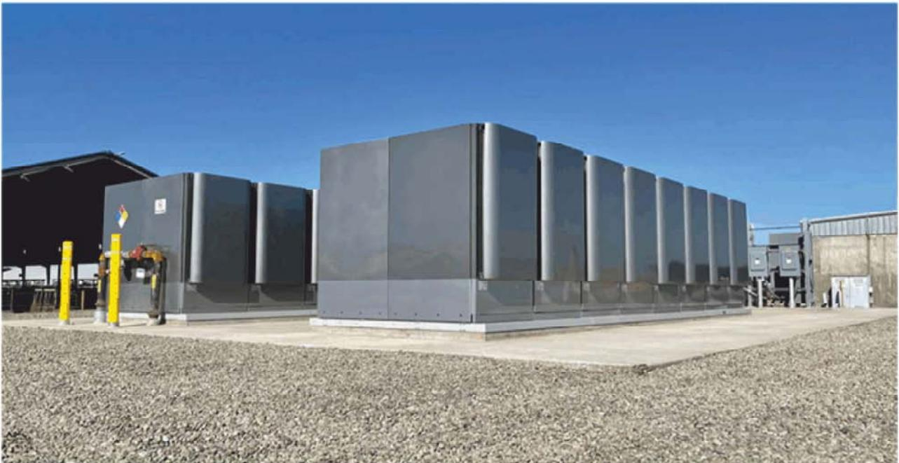
Bloom Energy Corporation (Bloom Energy) has announced the deployment of a 1 MW fuel cell at Bar 20 Dairy Farms in Kerman, California (CA) to efficiently produce on-site, renewable electricity from dairy cow manure. The installation marks Bloom's first dairy farm biogas project. Bar 20 Dairy Farms combined a methane digester, gas clean-up skid, and Bloom Energy fuel cells for an end-to-end, waste-to-electricity solution (photo courtesy Bloom Energy).
